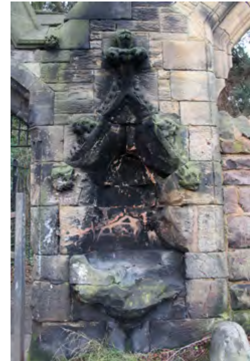
There is evidence of the water fountain on the external wall of the gate. Note the vandalism and fire damage.
