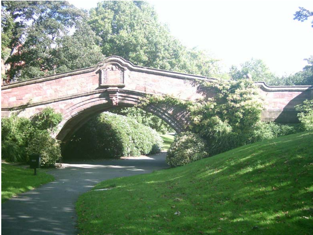
Photograph 3 View of bridge facing north-east
