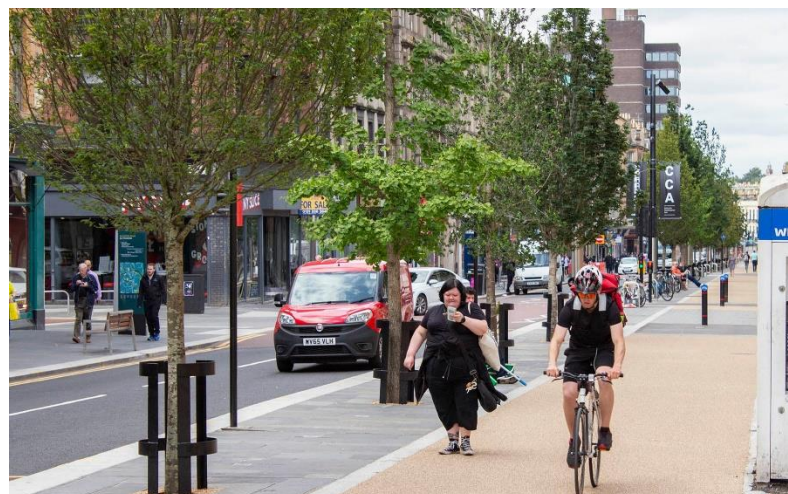
Bi-directional segregated cycleway and tree planting Sauchiehall Street, Glasgow
